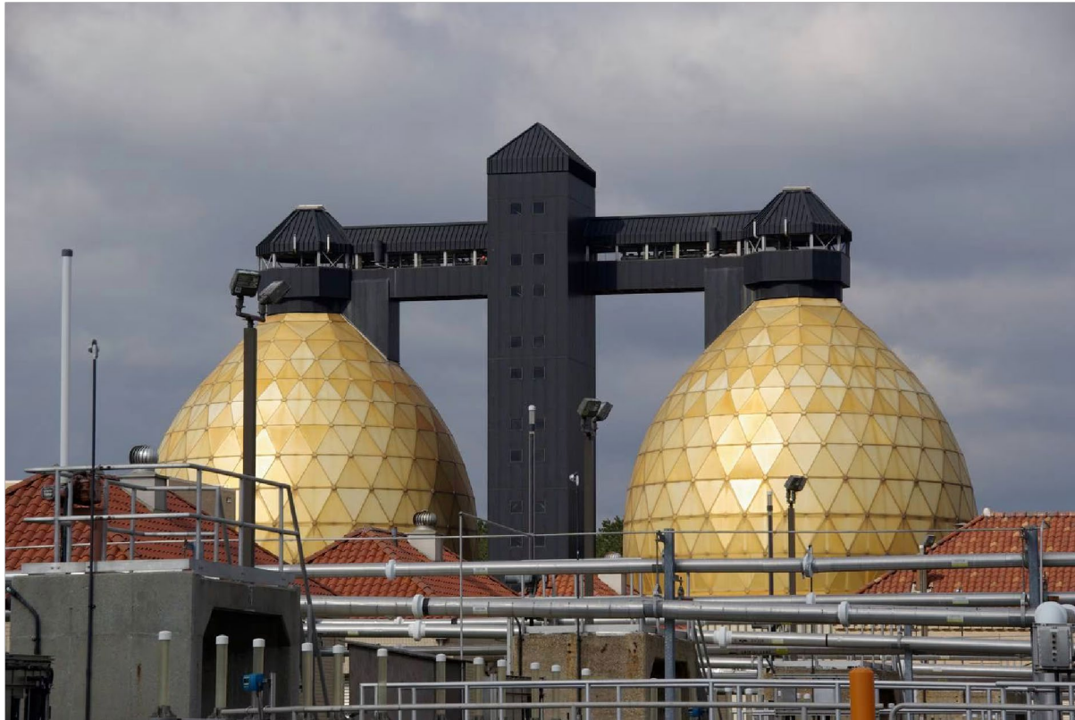
The two digesters at the Back River Wastewater Treatment Plant near Baltimore. (Kristian Bjornard/Wikimedia Commons)
