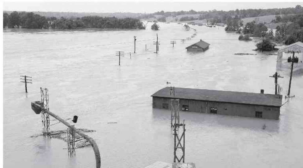
A post-Agnes view of Cartersville, VA, on the James River about 25 miles west of Richmond. The flood destroyed the Route 45 Cartersville Bridge, built in 1884, carrying away its four center spans. The two shoreside spans of the bridge still stand beside a new bridge and are preserved as historical sites. (Library of Virginia via Flickr Commons)
