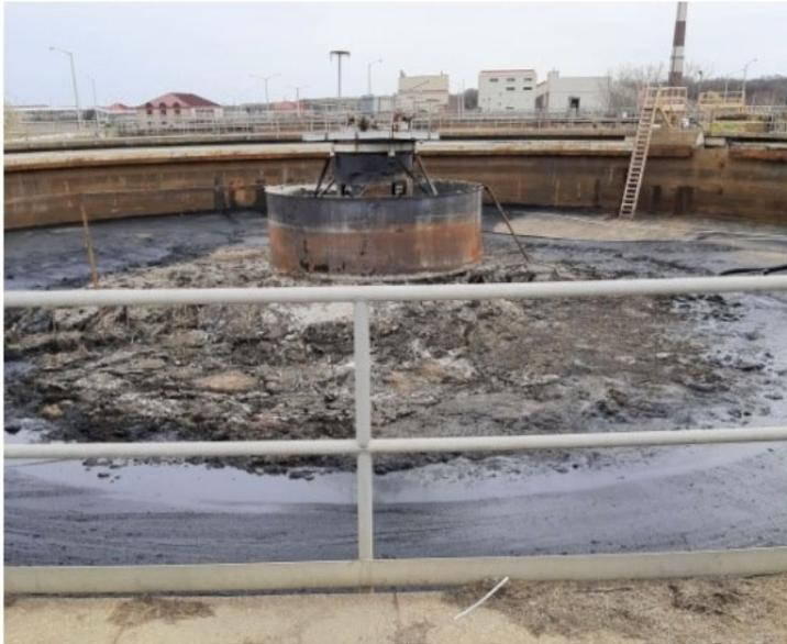
An inoperable settling tank clogged with hardened sediment at Back River. (3/22/22 inspection by MDE)
