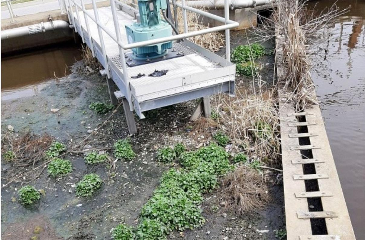
Solids buildup with vegetation growing in the biological reactor found during the March 22 inspection of the Back River Plant. (MDE)
