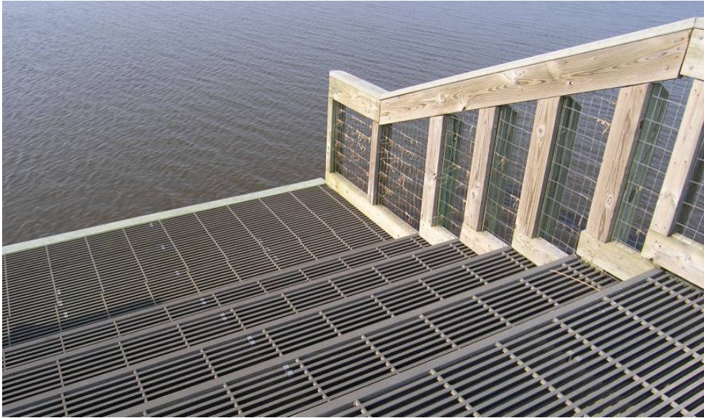
Figure 30 – A fixed dock with steps descending into the water for launching is difficult for users with mobility handicaps
