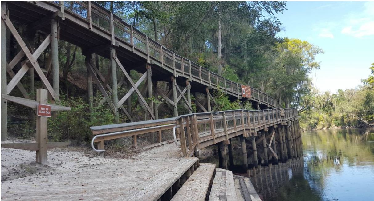
Figure 28 – Though ADA accessibility is provided to the launch point, the stairs become an impediment for users with handicaps
