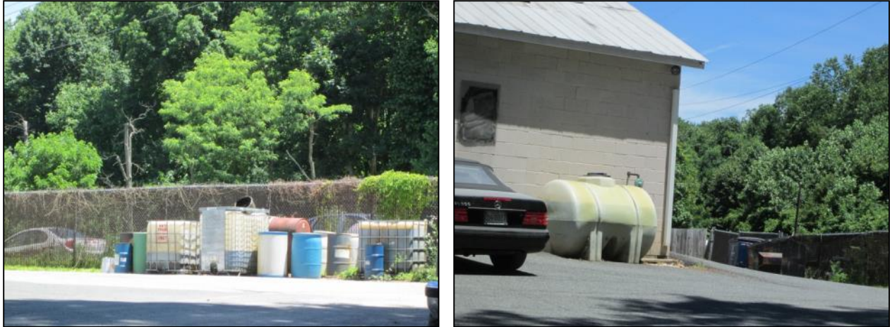
Figure 4-10: Outdoor material storage without secondary containment as HSI_G_402
